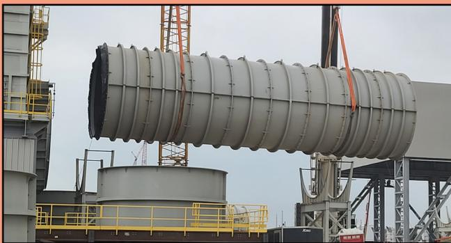
Adelphi Construction LC completed the installation of 22' diameter ductwork alongside IAC auxiliary baghouses on site at Steel Dynamics Inc's new melt shop being constructed in Sinton, TX.
