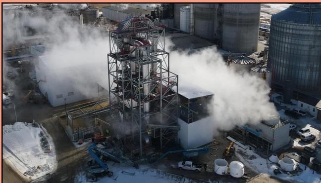
Adelphi Construction LC recently supplied structural steel and staircases for this Ethanol Plant project, plus provided specialty construction trade services to install a ring dryer and other process equipment including vertical centrifuges, horizontal decanters, pressure gravity screens, drag and screw conveyors, tanks, agitators, scrubber with internal packing, centrifugal pumps with seal pots, and a track operated building hoist. All work was performed during a time sensitive plant shutdown.
